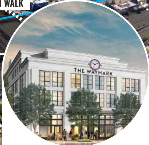
The Walnut Creek Transit Village is a mixed-use development recently completed at the Walnut Creek BART Station. The Village contains 358 "Class A" apartment units, 14,000 SF of shops and restaurants with outdoor areas designed for dining, views to Mt. Diablo and direct pedestrian access to BART.
